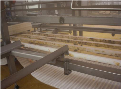
Figure 7. Wear strip dirt detected after the conveyor belt has been dismantled
