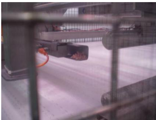
Figure 8. Remained debris in a U-profile
